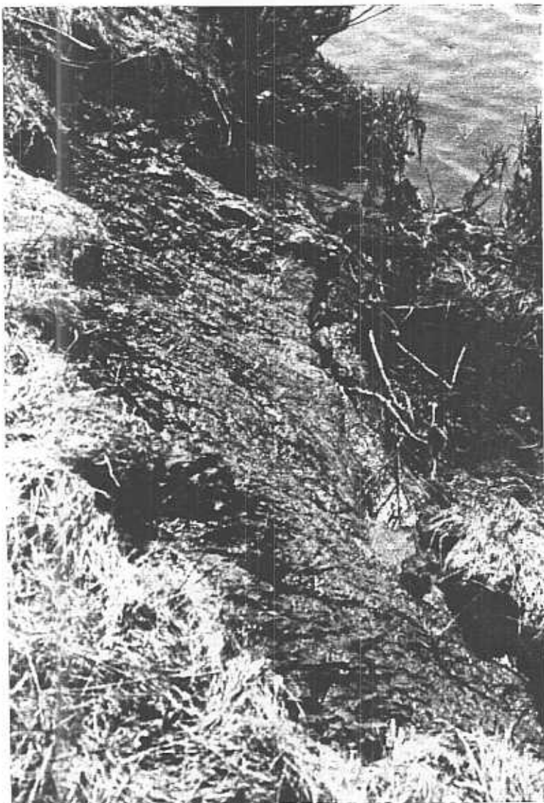
Figure 2.2 Landslip at Fort Anne, March 1994. High Water.
