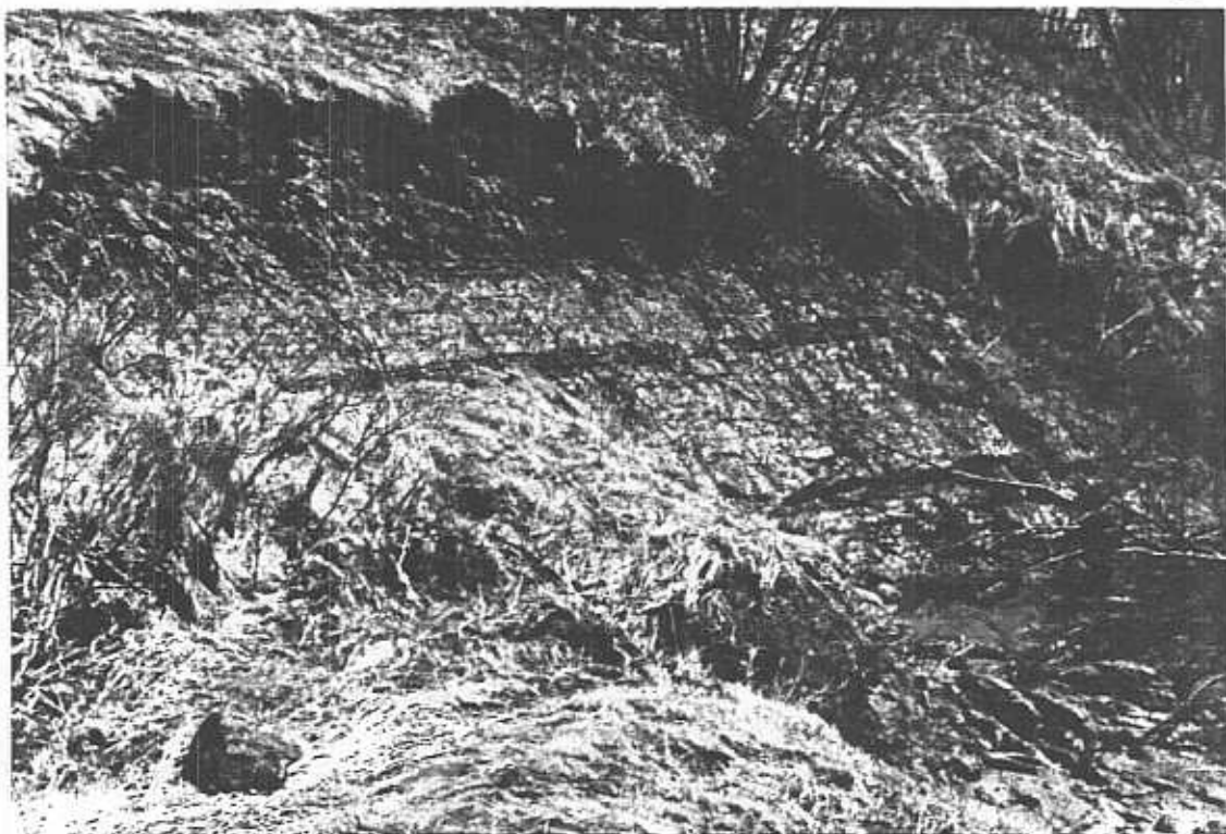
Figure 2.1. Landslip at Fort Anne, March 1994
